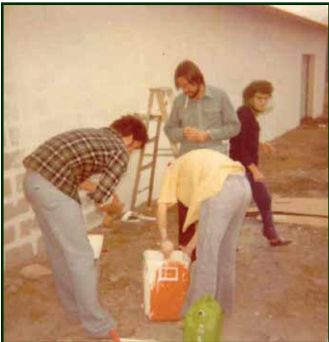
The first coat of paint was brushed and rolled on the new DTCCD building in 1975.
