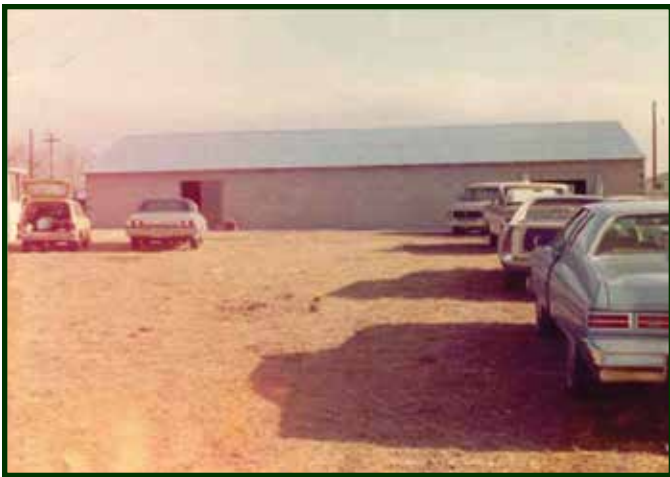
Walls, roof and floor were completed by December 1975; the first weekend of December club members turned out and installed electricity and applied paint – and classes were held in the new training building in the first week of December.
